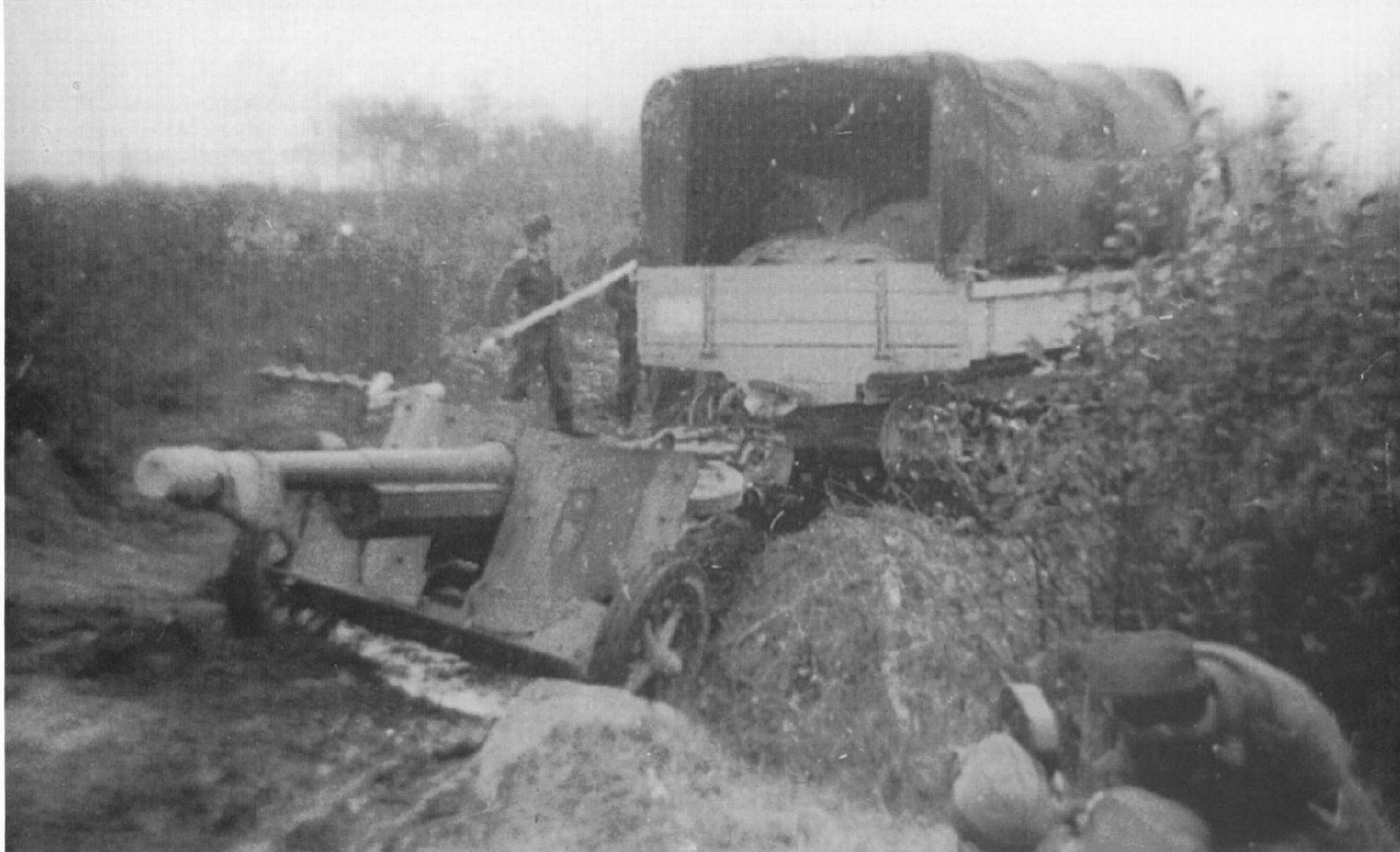
The 7.5 cm Antitank Gun 97/38 shows that antitank troops needed to obtain better weapons as fast as possible in 1942. The barrels of numerous captured French mle. 1897 Cannons were installed in the mounts of the 5 cm Antitank Cannon 38. At first, ammunition captured from Poland and France was used. With the German-made 7.5 cm 97/38 HL B (f) shell, armor 75 mm thick could be penetrated. In all, 860 97/38 Antitank Cannons were made.
