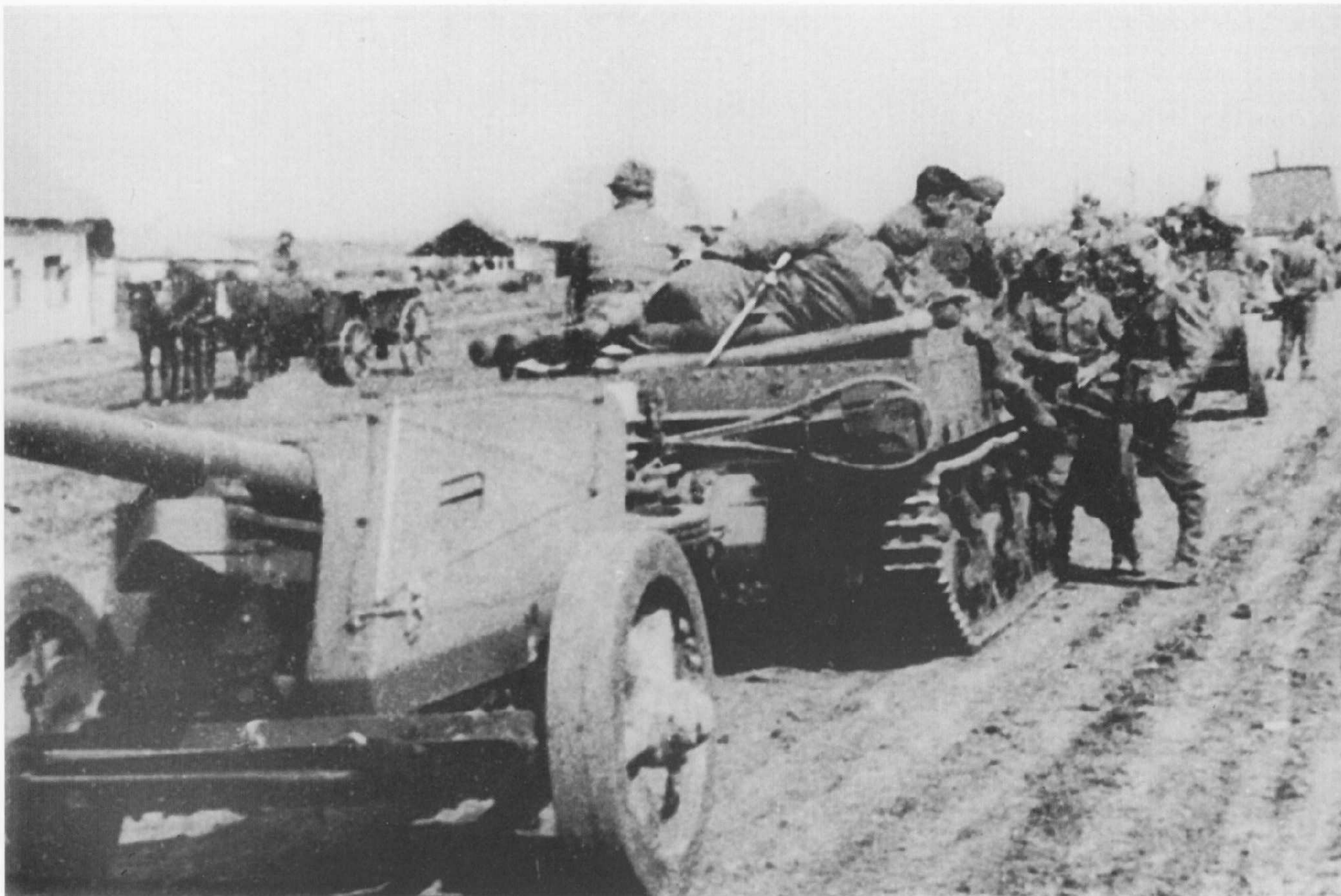
In the spring of 1942, the Army tried particularly to make the Panzerjäger units deployed on the southern part of the eastern front more mobile by issuing them towing vehicles. This picture, taken in the 14th Panzer Division's sector in June 1942, shows a MK II 603 (3) light artillery tractor towing a 7.5 cm Antitank Gun 40 L/46.
