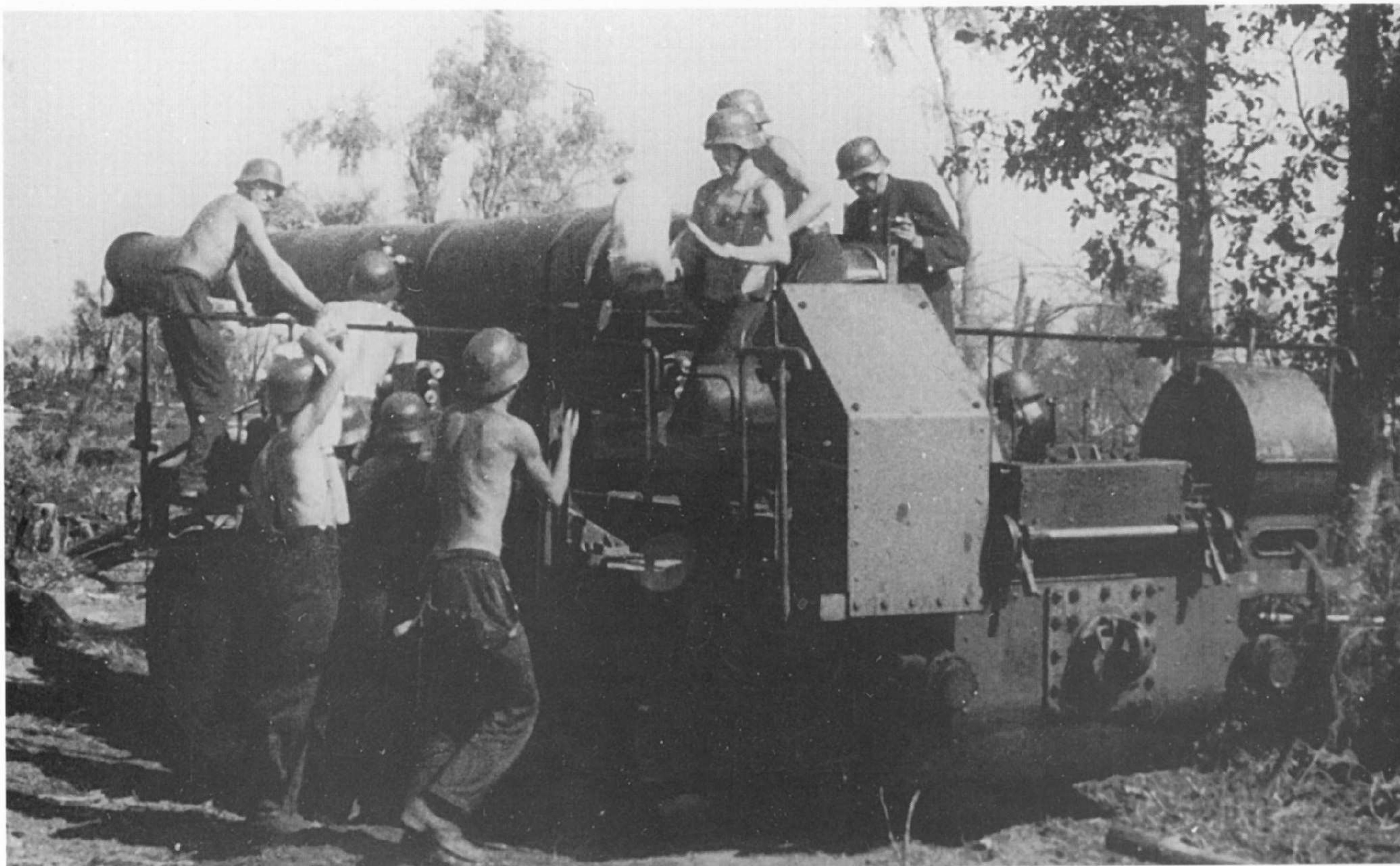
A 19.4 cm Cannon 485 (f)-frz. GPF- in firing position on a self-propelled mount. The generator vehicle has been uncoupled and the gun car lowered. One gunner is handing a bag cartridge up to the work stage. The picture was taken in the summer of 1942 in the II. Unit, Army Artillery Regiment 84, in the northern sector of the eastern front.
